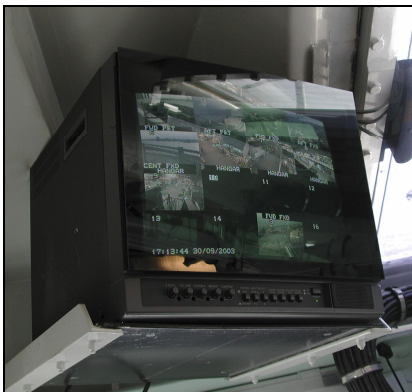
External filter retrofitted to warship display
